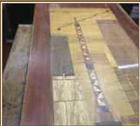
Finally fitted and fixed in place
