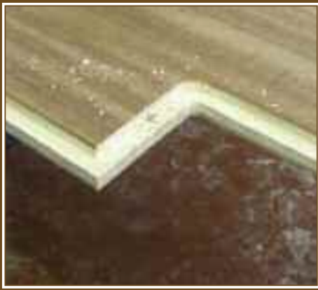
A nice example of clean routing
