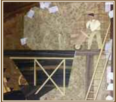
Ladder and supports added to insert
