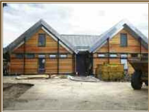
The New Hall nearing completion
