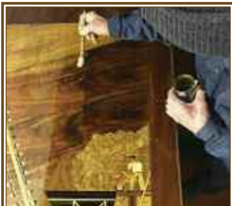
Applying the first coat of finish
